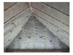
Fiberglass insulation can also be installed to comparable densities, although is typically subject to the same vulnerabilities as noted above. Spray fiberglass is becoming increasingly available, with fibers typically mixed with acrylic bonding agent.
